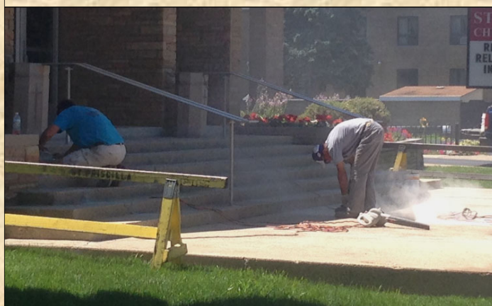
This picture shows some workers repairing the cracks in the sidewalk and steps of the main entrance to the church.
