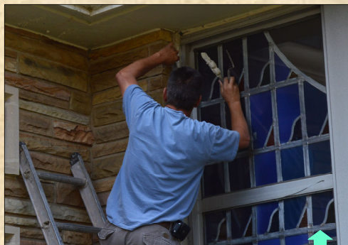
This is a picture showing a worker caulking the southside window in the vestibule of our church.
