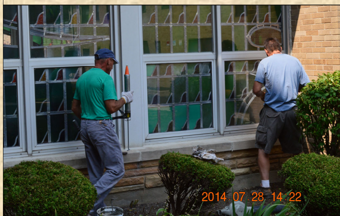
Here we see two workers repairing the southside window by putting on new caulking.
