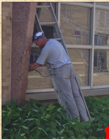
Another worker caulking the east wing big window of our church.
